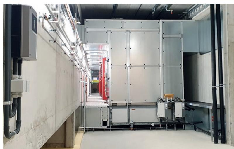
The technological double-act at this data centre in eastern Switzerland shows the scalability of the ServeCool solution. There are already five devices installed, out of a possible eight if the system were to be extended over the full area the ground floor.
