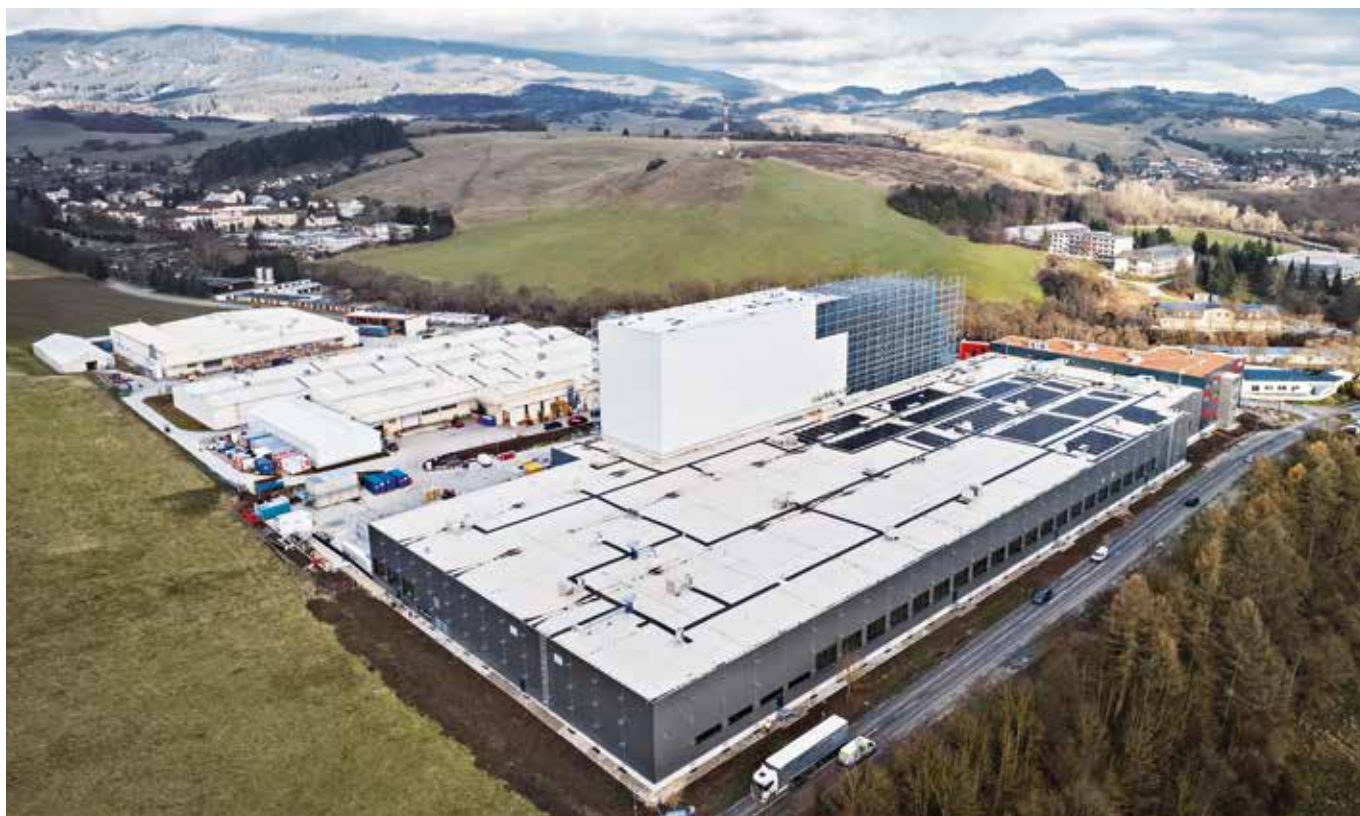
Hoval is building a new state-of-the-art heat pump factory directly adjacent to its existing factory in Istebné (Slovakia). It will commence operation in 2025.
